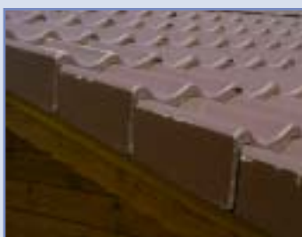
Beton/Tonziegel mit/ohne Organg
